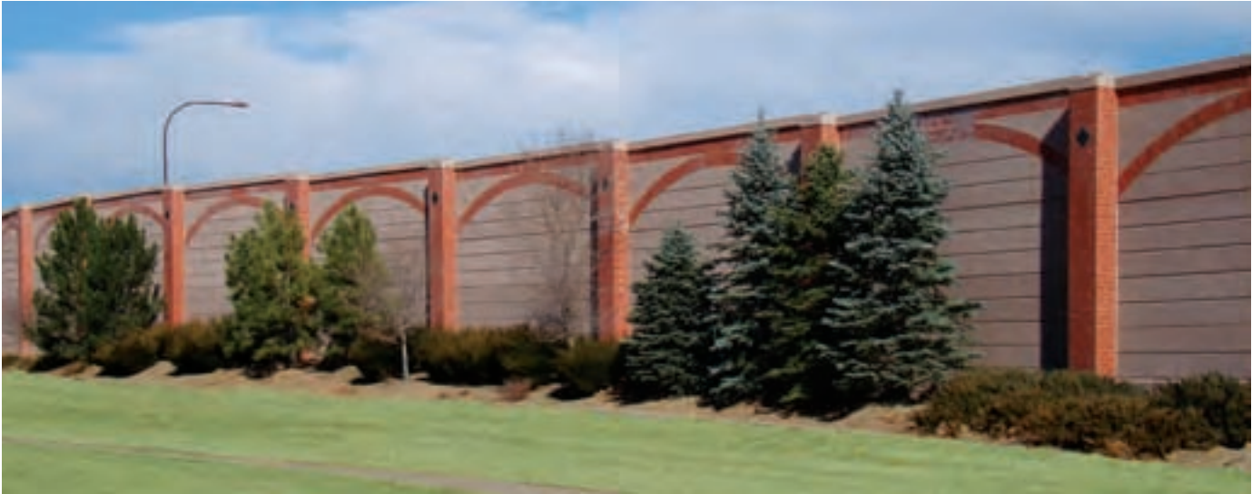
Thin Brick and Stone Vertically Embedded in Concrete
