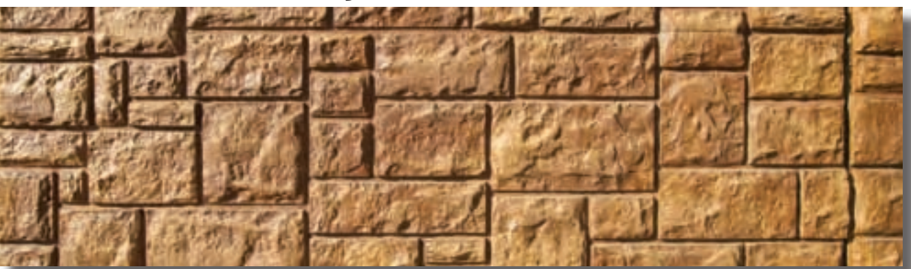
Ashlar panels abut, creating vertical and horizontal joints. To the passerby, what appears to be a wall is actually a series of concrete panels coming together with Scott form liner. Can you see the panel joints?
