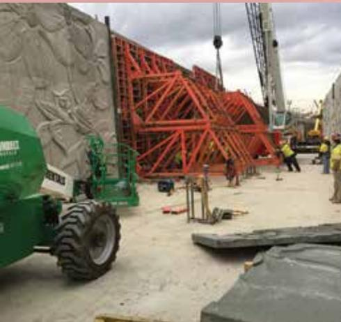
Scott System's elastomeric form liners are attached to large concrete forms used to pour the retaining walls approaching the tunnel.
