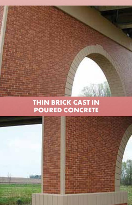
Highway and bridge departments are specifying poured-in-place concrete walls with integrally cast brick, thanks to the patented Rim Snaps™ system. Minnesota and Wisconsin DOT's have constructed a number of projects featuring brick-embedded concrete.
