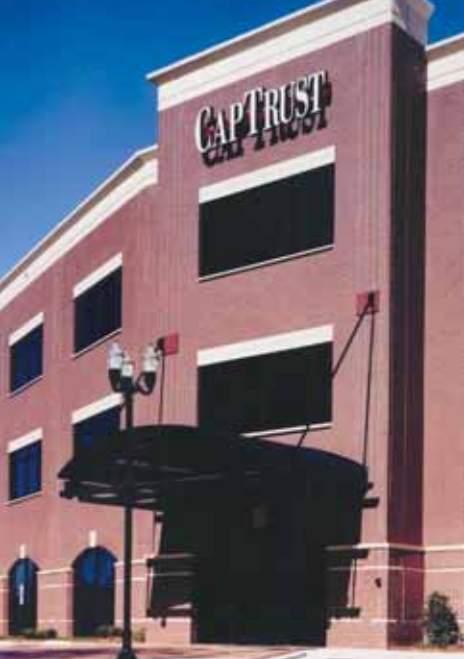
Beacon Center Office, Raleigh, NC Centurion Construction, Raleigh NC
