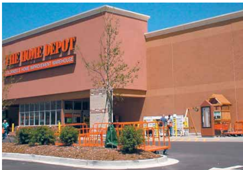
Home Depot, Denver, CO Colorado Structures, Colorado Springs, CO
