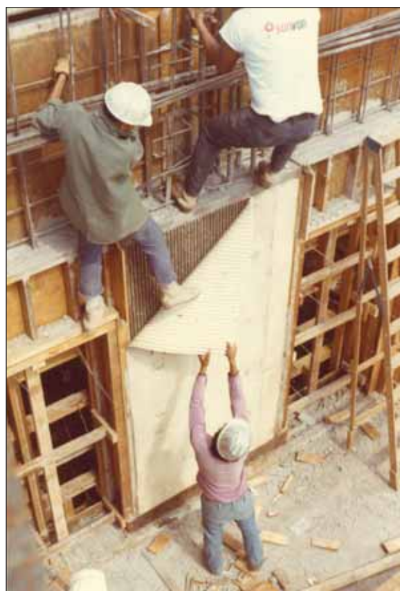
One of our first Flex-Liner™ textures, Fractured Fin was made in white urethane elastomer back in 1971. Here contractors strip the liner in their own creative way.
