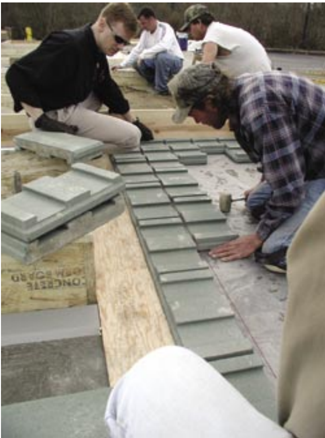
One thin block system, Chameleon Cast Wall, an embedded masonry option, can offer special design patterns, including mosaics or tiling, without complicating a construction schedule
