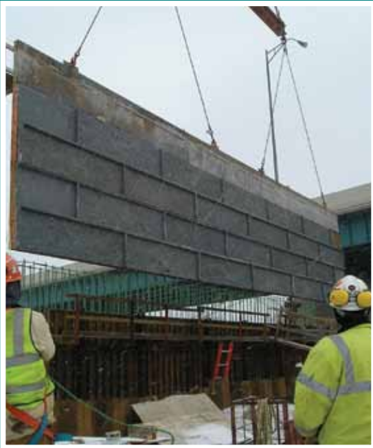
Kokosing Construction uses Scott System elastomeric form liner molds to recreate the old-time railroad bridge piers seen in the background.
