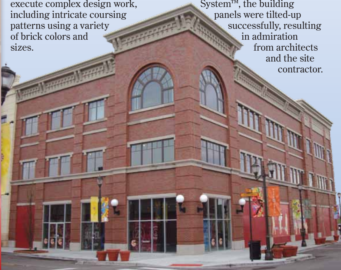
Buildings were constructed with cast-on-site load bearing wall panels. Because of tight site conditions, cranes were positioned on adjacent streets and panel erection was performed at night to avoid foot traffic.
