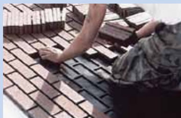
In 1991, Scott's Snap System had yet to be invented, so the elastomeric brick gasket liner was used to hold brick in place.
