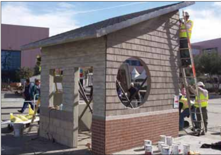
World of concrete Mega-Demo featured many exterior options for concrete including a scallop-pattern roof, cedar and shake textures, stone and brick-embedded concrete and paint finishes.
