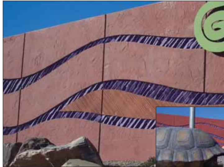
"Spaghetti Bowl" (Intersections I-15, I-515 & US-95) in Las Vegas, NV was designed with a flowing wave of color and texture combining three Scott System patterns: Rocky Mountain Flagstone, Oregon Basalt and Striated. Project team includes Zunino Engineering, NDOT and Capriati Construction, Las Vegas, NV.
