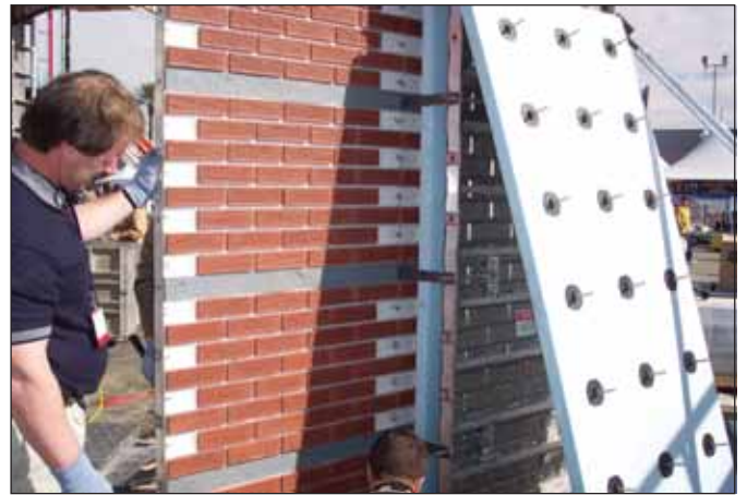
Rim Snaps and Flagstone form liner are placed on Durand forms, followed by the Thermomass® insulation system.
