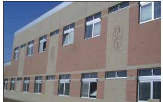
An elementary school in the new Stapleton Development of Denver incorporated decorative precast concrete into the building exterior. Elements include 3 1/2' x 6' medallions representing school subjects like reading, math and art. A planter/bench in the main entrance area features the earth strata and fossils. Design by Gavin Woodsworth of Norris Design, Denver. Construction by IFC Constructors and precast by Rocky Mountain Prestress.
