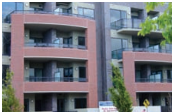
The Santorini Apartment complex in Melbourne, Australia is an excellent example of a high-rise precast housing structure with brick-embedding concrete. Photo courtesy of Daniel Robertson Ltd., Melbourne.
