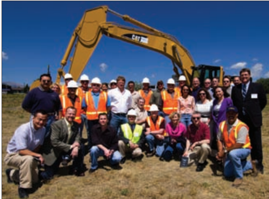
SEMA's team ready to break ground on Colorado Springs' COSMIX highway project.
