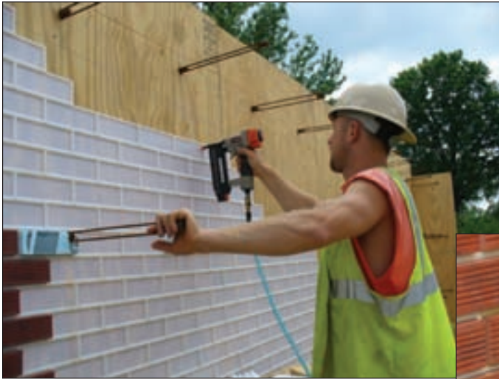
Above: Rim Snaps™ are attached to vertical forms with staples. Brick is inserted into the templates and form ties are set. A foam blockout fills the brick pocket to accommodate the form tie. A thin-set brick patch fills in after the forms are removed.
