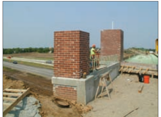
Above: A worker details a brick column on the Valley Creek project. This is a fast track construction job on the six-lane bridge that spans over Interstate 494 east of the Twin Cities.
