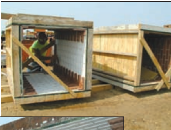
Above: A worker details a brick column on the Valley Creek project. This is a fast track construction job on the six-lane bridge that spans over Interstate 494 east of the Twin Cities.
