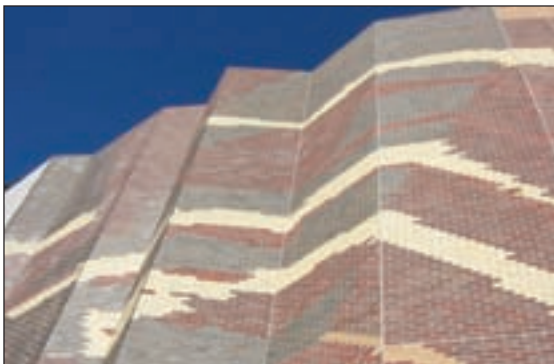
Above: In addition to slanting the brick patterns, H2O Architects' design utilized precast panels set at varying angles.
