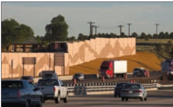
Colorado Springs Metro Interstate Expansion (COSMIX) includes precast concrete panels with patterns suggesting the Rocky Mountains.
