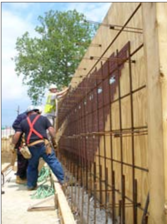
Above: Rim Snaps™ are attached to vertical forms with staples. Brick is inserted into the templates and form ties are set. A foam blockout fills the brick pocket to accommodate the form tie. A thin-set brick patch fills in after the forms are removed.
