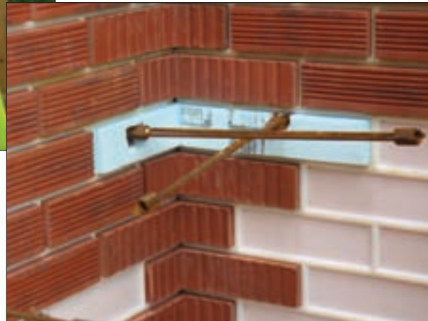
Left: Brick, ties and rebar are set. Workers make final adjustments before closing up the form.
