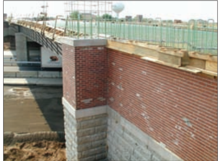
Above: The Valley Creek Bridge in Woodbury, MN features a blend of brick with a hand-crafted finish on piers and abutments. A limestone base created with form liners complete the traditional design. Brick will be thin-set in the voids where form ties were located. Then remaining concrete residue will be washed off.
