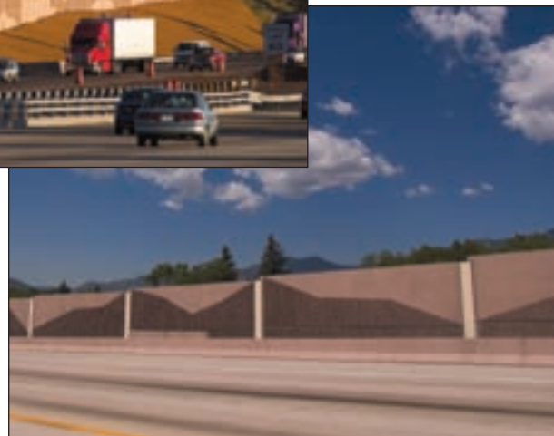
Colorado Springs Metro Interstate Expansion (COSMIX) includes precast concrete panels with patterns suggesting the Rocky Mountains.
