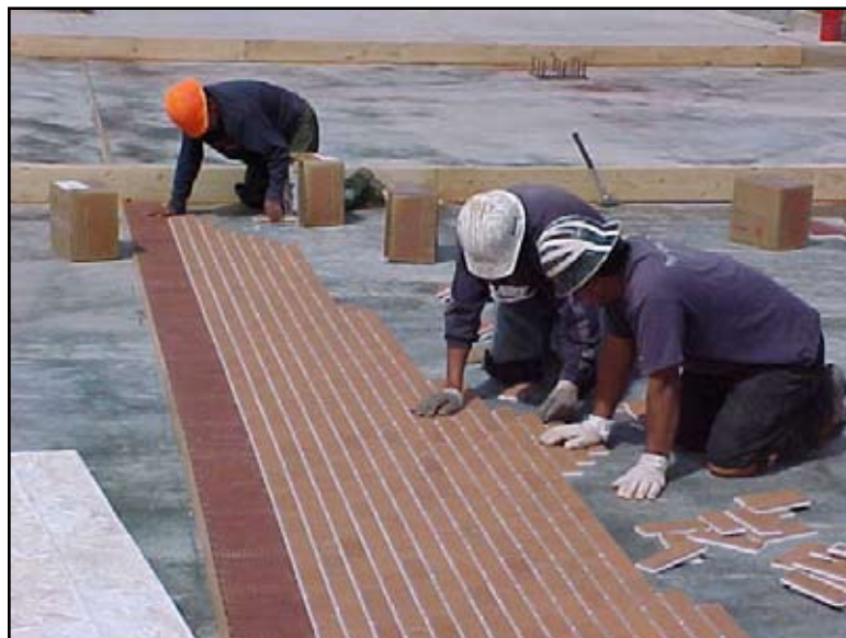
Brick snaps together at a rate of 50-60 sq. ft. per man hour.
